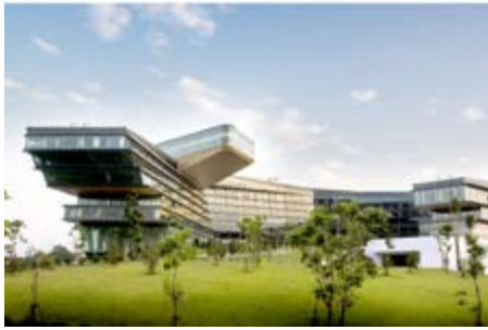
Artu switchboards, breaker & switches, DIN-RAIL products, control products at JW Marriott Hanoi Hotel
