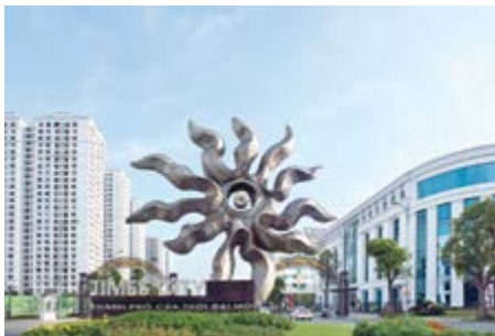
Breaker & switches, DIN-RAIL products, control products at Times City
