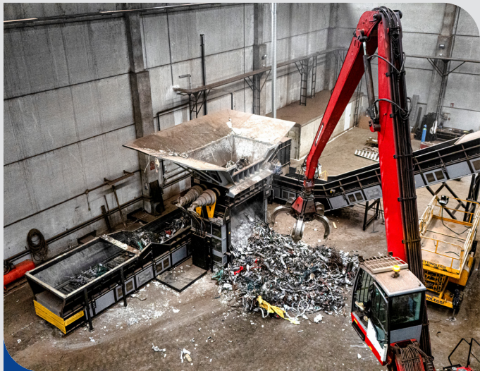
Proler production plant
