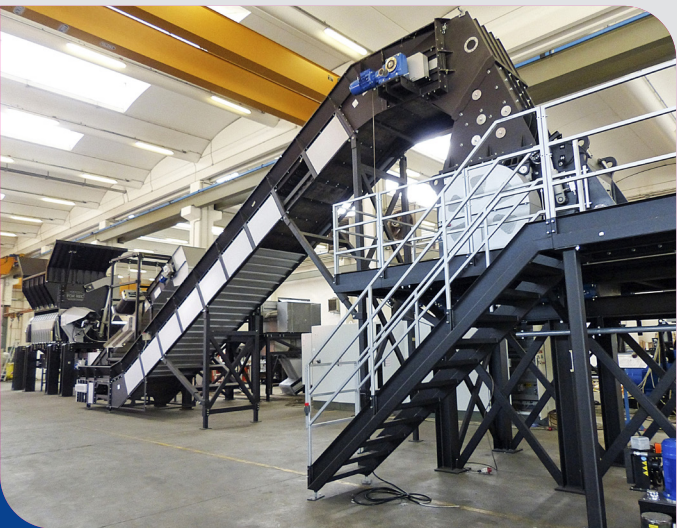
Aluminum Scrap Treatment Plant
