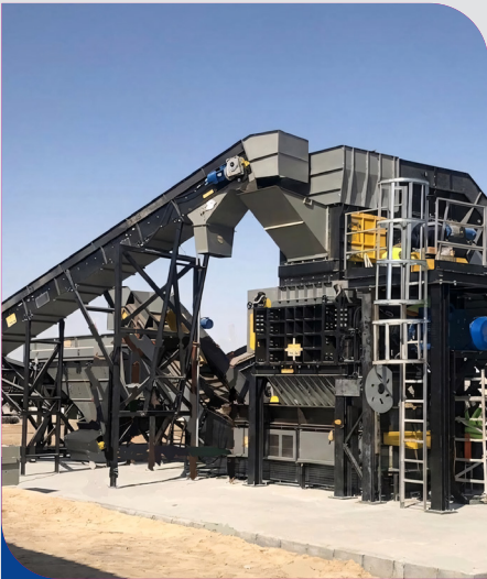
Chip production plant (20 × 20 mm)
